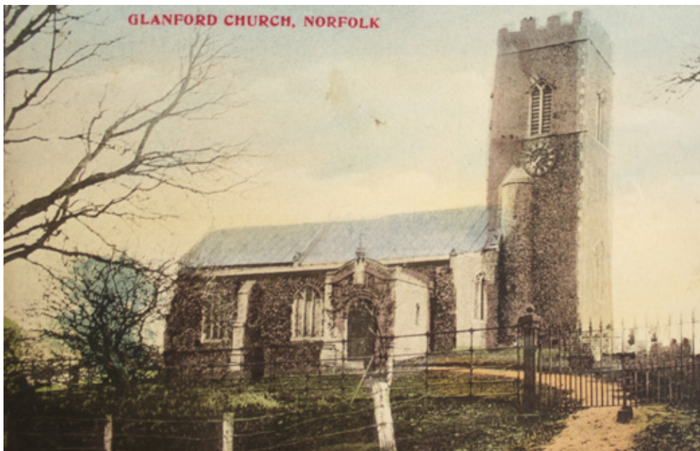
View of Glandford Church showing the iron boundary fencing, which remains in part today (Norfolk Record Office: C/GLA)
