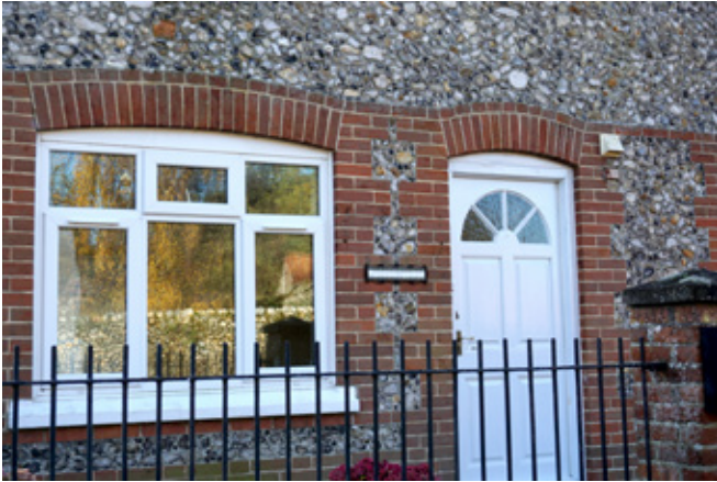
uPVC window and modern replacement door
