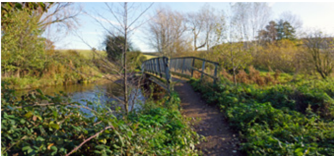
The bridge over the ford
